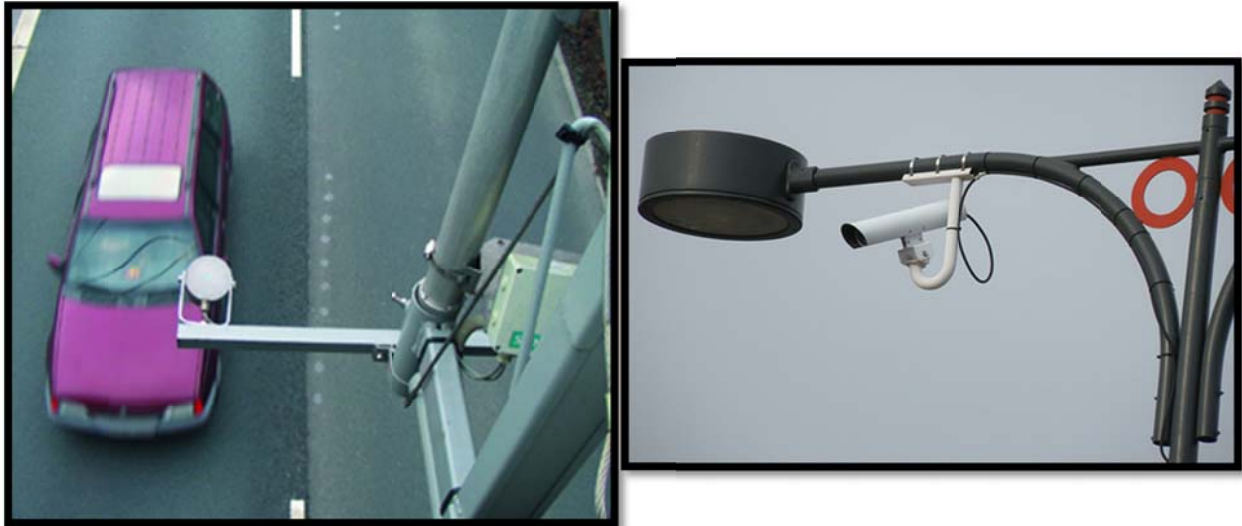
Figure 5-4 Photographs showing the installation of video capture devices installed in the field 24,25
